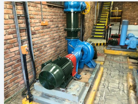
MOTOR-DRIVEN CENTRIFUGAL PUMP INSTALLATION
