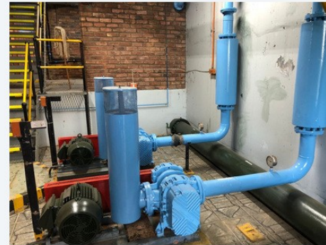
TWIN PUMP INSTALLATION AND DISCHARGE PIPEWORK
