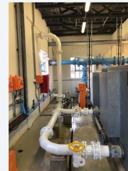
PLANT-ROOM PIPELINE INSTALLATION
