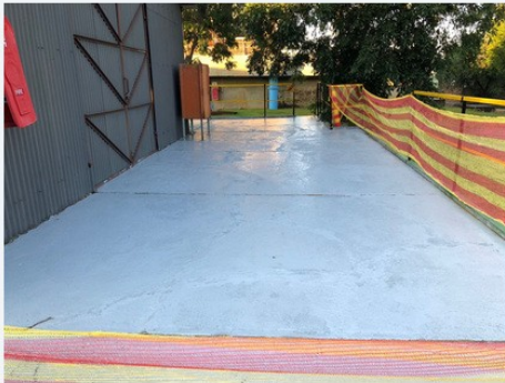
FINISHED CIVIL FLOOR AND ACCESS AREA
