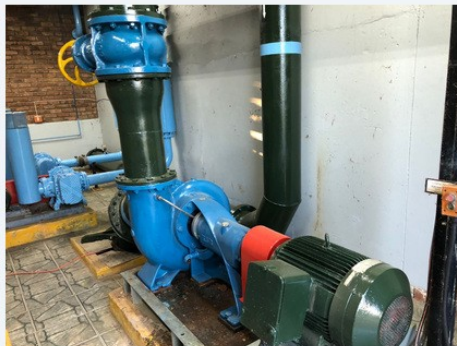
PUMP AND MOTOR INSTALLATION
