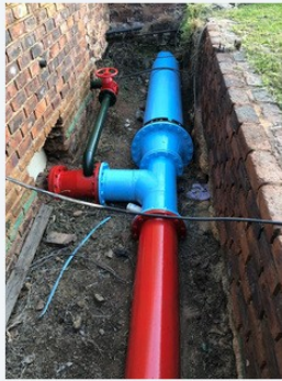
LARGE-DIAMETER PIPEWORK AND VALVE INSTALLATION
